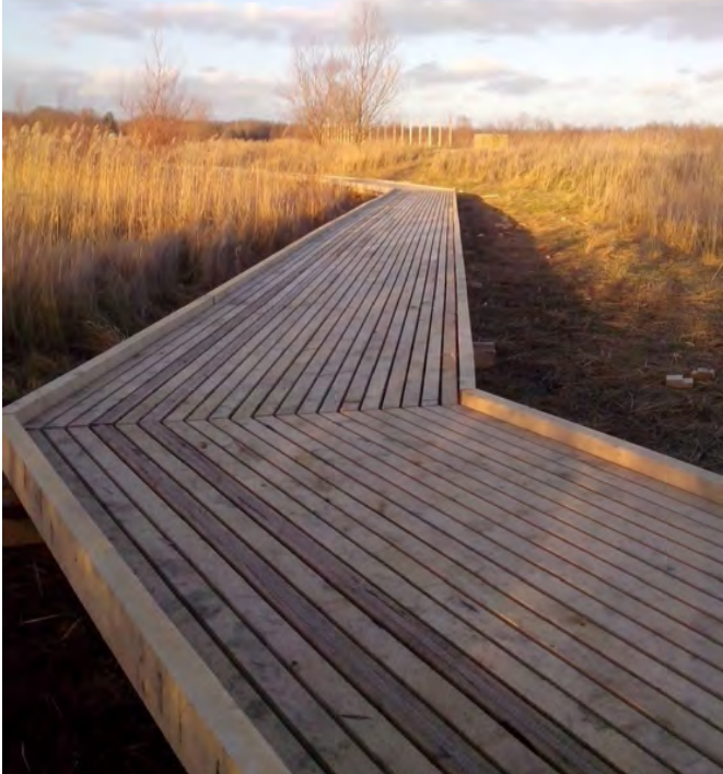
ACCESSIBLE ROUTE BOARDWALK
