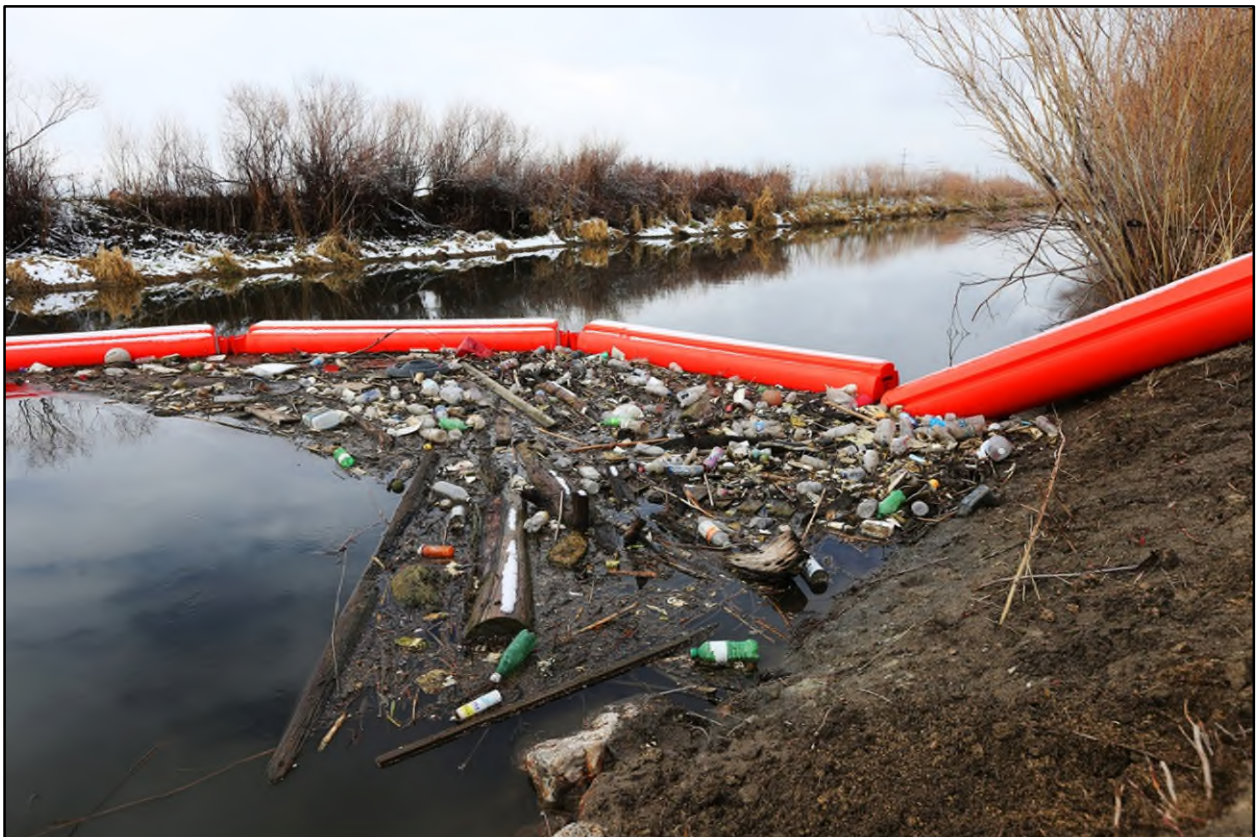
Figure 5-4. Trash boom installed on the Jordan River (KSL News 2018).
