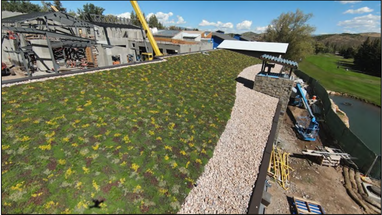
Figure 5-3. Green roof installation at 3 Kings Water Treatment Plant in Park City, Utah (Intermountain Roofscape Supply 2025).
