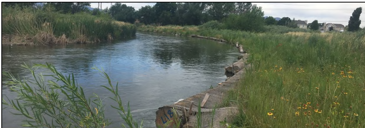
Figure 5-6. Streambank restoration project (Salt Lake County 2025d).
