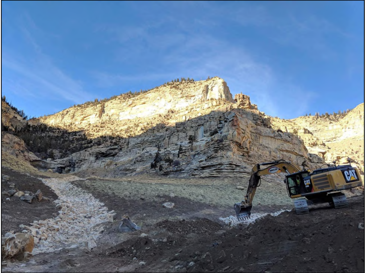
Figure 5-5. Cottonwood Mine reclamation project in Emery County, Utah (WW Clyde 2018).
